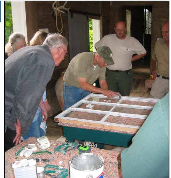
Historic windows are among the most important elements of a building. Simple repairs and routine maintenance coupled with storm windows make for energy efficiency that in most cases matches, if not exceeds, the efficiency of replacement windows. Workshops throughout the region have taught building owners easy ways to care for their historic windows. At the Woodlawn Museum in Ellsworth, ME, a grant from the National Trust for Historic Preservation helped fund a window repair workshop. Photo courtesy of the Woodlawn Museum
