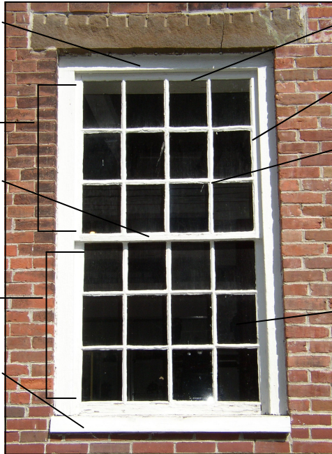
A c. 1846 wood window in the former Robbins and Lawrence Armory, now the American Precision Museum in Windsor, VT.
