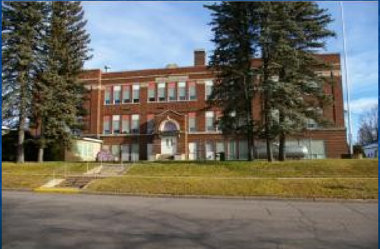
Lincoln Elementary, soon to be Lincoln School Apartments Park Falls, WI
